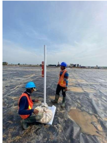
Gambar 2.30 Settlement Plate (Sumber: PT Geostucture Dynamics, 2023)
