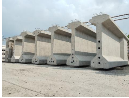
Gambar 2.7 PCI Girder Segmental
