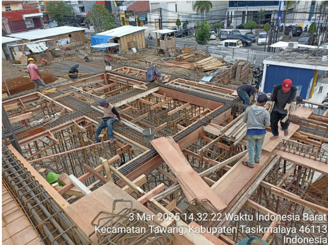
Gambar 3.21 Bekisting Balok
