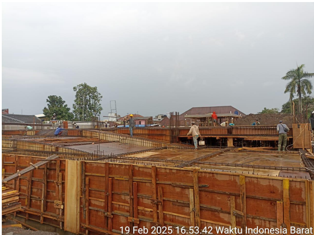
Gambar 3.20 Bekisting Dinding Basement
