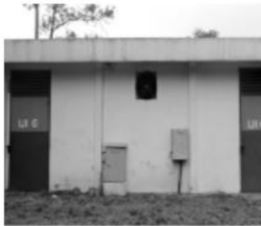
Gambar 2. 7 Gardu Beton
