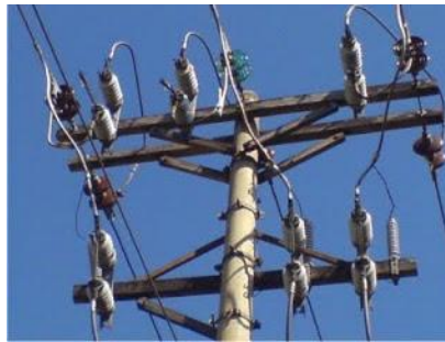
Gambar II. 14 Disconnecting Switch (Annisa & Mardiansah, 2023)
