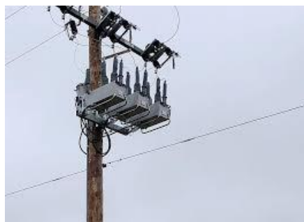
Gambar II. 16 Recloser (Gede Wiyoga Putra et al., 2020)
