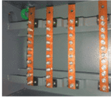
Gambar 2. 7 Busbar Panel
