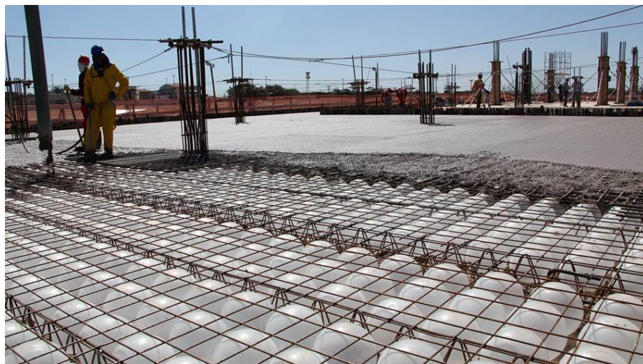
Gambar 2.8 Insitu Concrete Bubble deck
