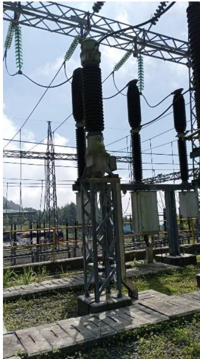
Gambar 2.4 Current Transformer Di PLTP PGE Area Karaha
