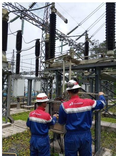
Gambar 2.9 PMT Three Pole Di PLTP PT.PGE Area Karaha
