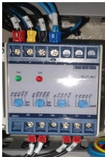
Gambar 2.15 Over Under Voltage Relai (OUVR)
