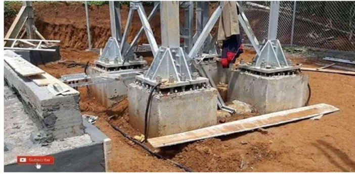
Gambar 2. 15 Pondasi Steel
