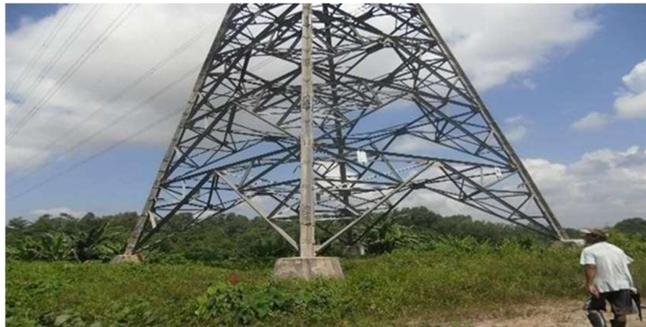
Gambar 2. 14 Pondasi Tower (Lattice)
