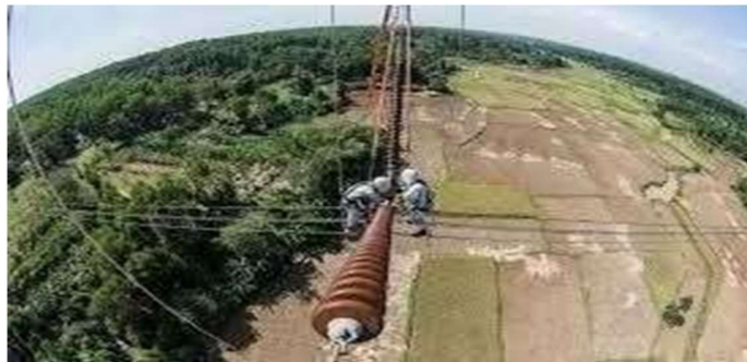
Gambar 2. 10 Ceramic Isolator
