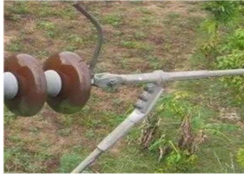
Gambar 2. 7 Jumper Point
