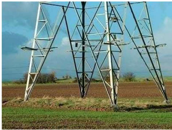
Gambar 2. 18 Anti Climbing Device
