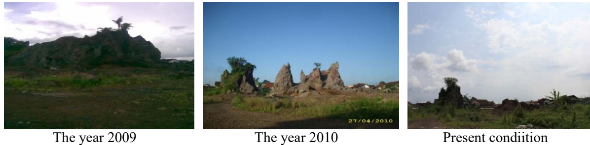
Figure 1. Development of Ten Thousand Hills Damage Level
