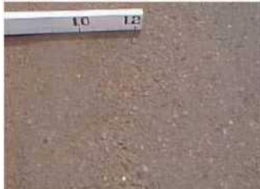
Gambar 2.12 Pengausan Agregat ( Polised Agregat ) Sumber : Bina marga no.03/MN/B/1983
