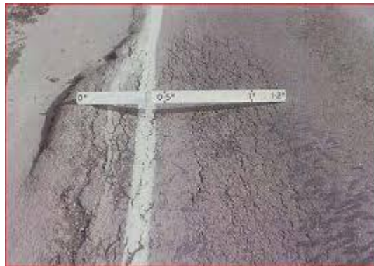
Gambar 2.16 Sungkur ( Shoving ) Sumber : Bina marga no.03/MN/B/1983
