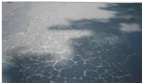
Gambar 2 19 Pelepasan Butir ( Weathering/Raveling )
