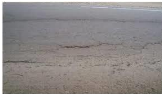
Gambar 2.4 Cekungan ( Bump and Sags )
