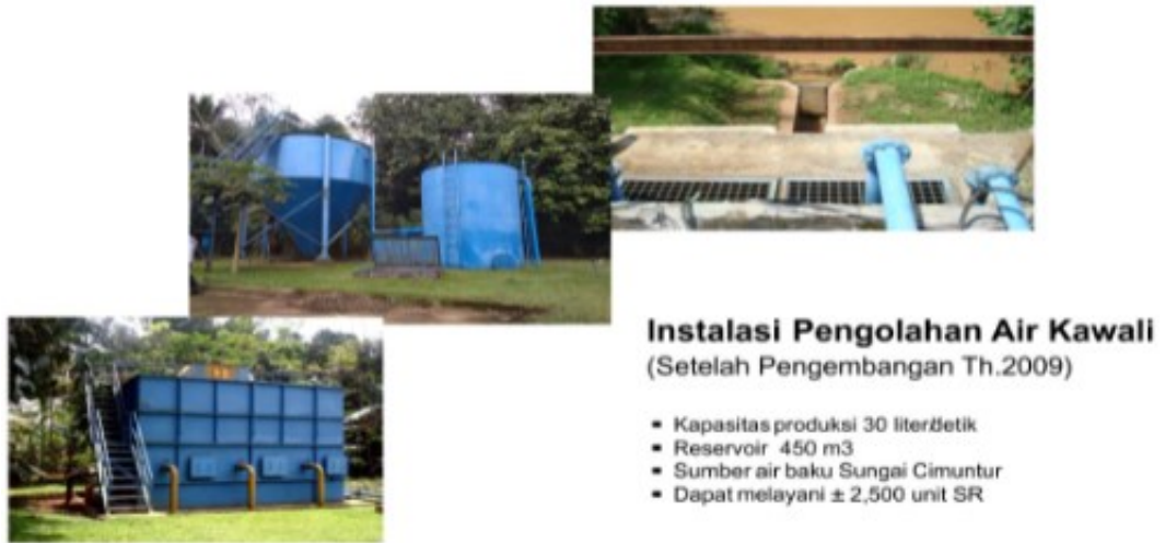
Gambar 3.2 IPA PDAM Tirta Galuh Ciamis Cabang Kawali (Sumber : PDAM Tirta Galuh Ciamis, 2020)
