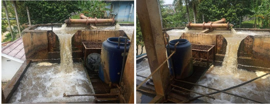
Gambar 2.10 Bak Koagulasi IPA Purwaharja PDAM Tirta Anom
