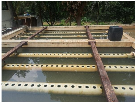
Gambar 2.12 Bak Sedimentasi IPA Purwaharja PDAM Tirta Anom
