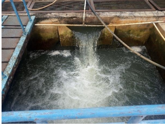
Gambar 2.13 Bak Filtrasi IPA Purwaharja PDAM Tirta Anom
