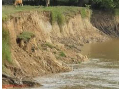
Gambar 2.9 Erosi Tebing Sungai
