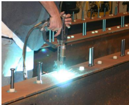
Gambar 2.32 Shear Connector
