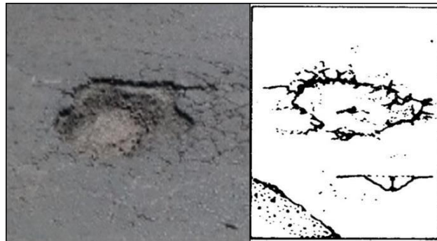
Gambar 2.22 Lubang ( potholes )
