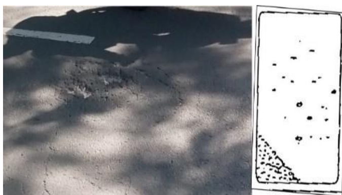
Gambar 2.39 Pelepasan Butir ( Raveling and Weathering )
