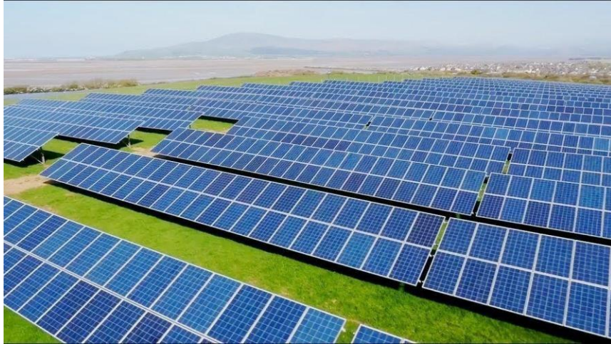
Gambar 2. 4 PLTS Ground-Mounted (ESDM, 2019)
